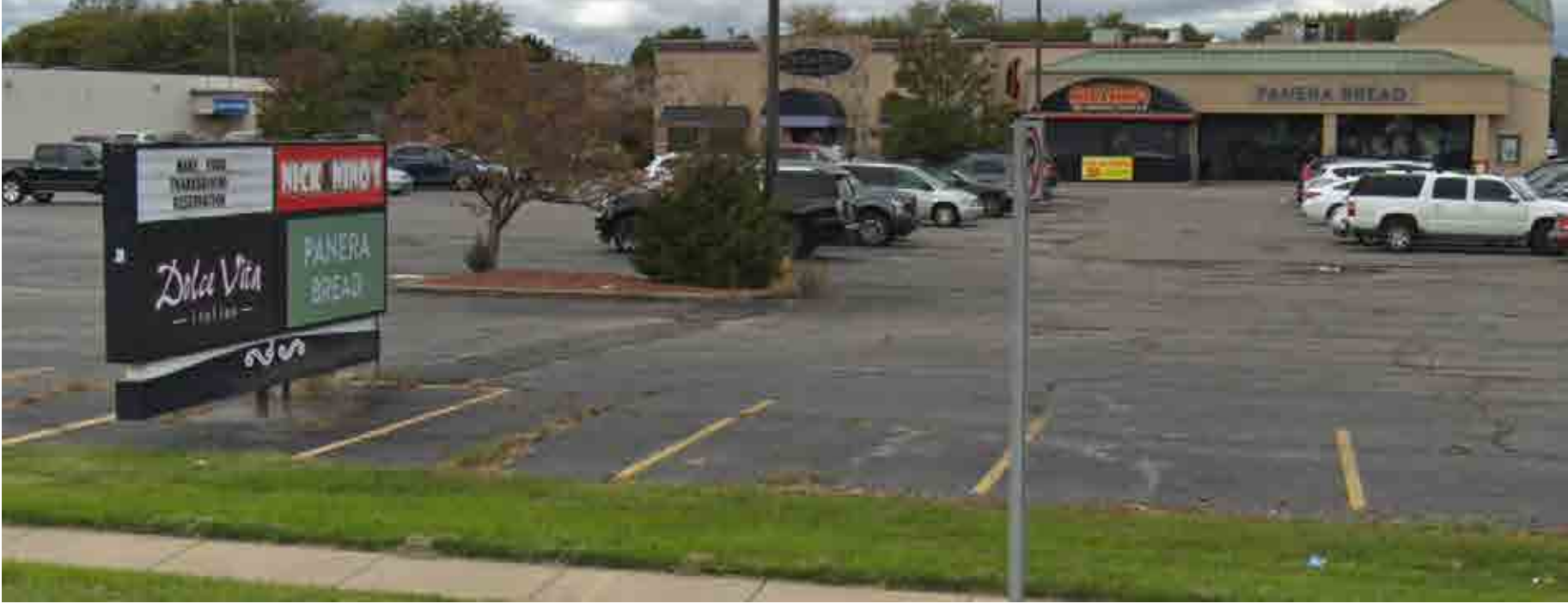
The Zoning Overlay should limit parking to the rear and/or side yards.
